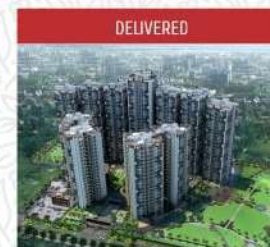
DELIVERED ACE ASPIRE 2/3 BHK APARTMENTS GREATER NOIDA (WEST)
